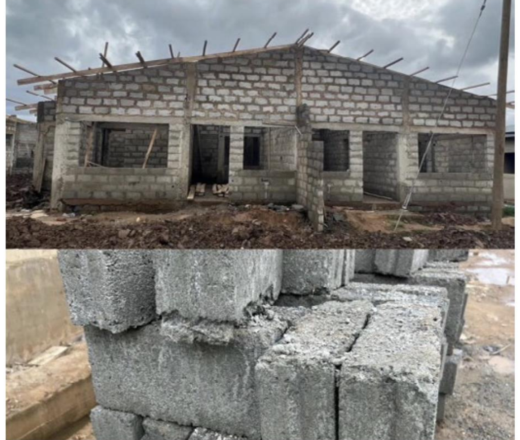
Traditional Block Construction:
